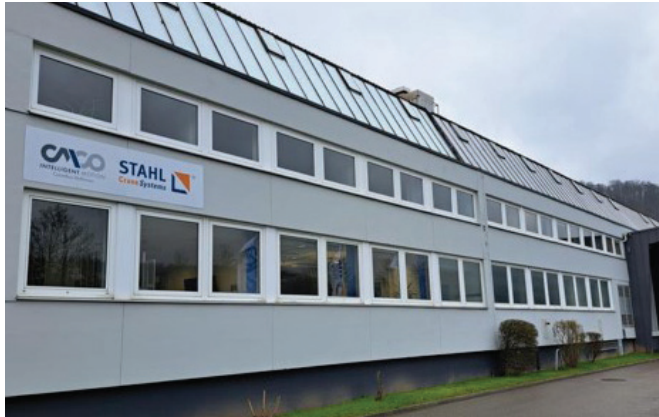
Building efficiency renovation projects
