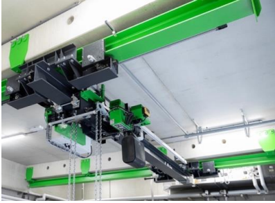
The crane runway mounted directly on the ceiling takes up very little space (Image source: Summer Metalltechnik)
